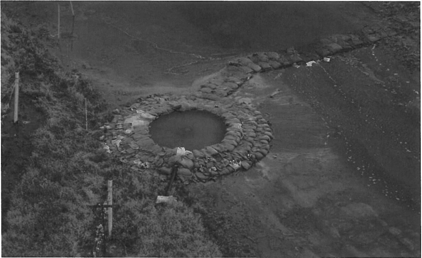
Sandbags temporarily control a sand boil on Staten Island on June 18, 2007. The muddy water indicates that material in the levee or its foundation is being washed away. Unnoticed, sand boils can lead to a failure of the levee. Source: DWR
