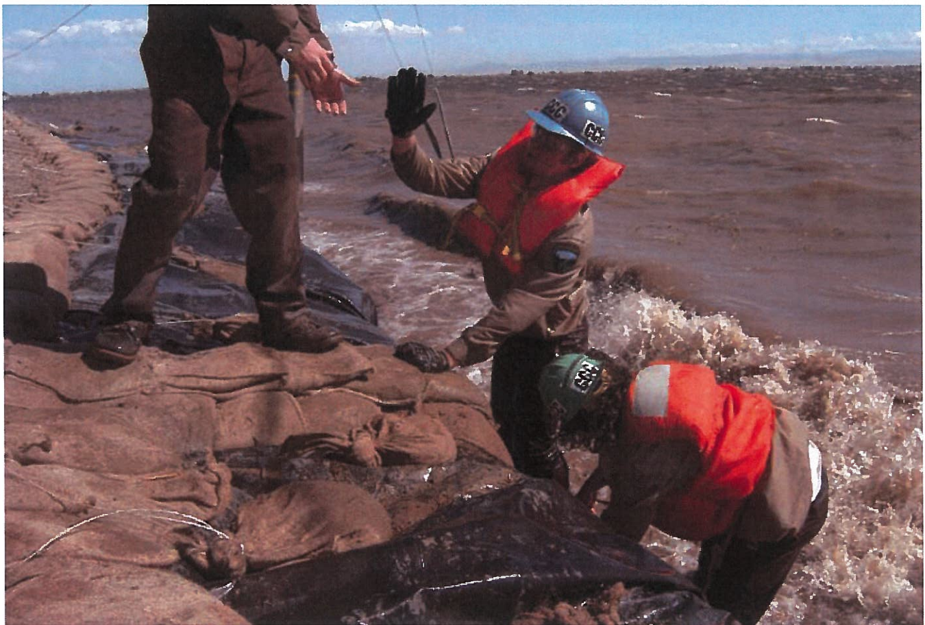
Pictured above: Protecting the land side of a levee on a flooded island [Upper Jones Tract, 2004]. Source: DWR
