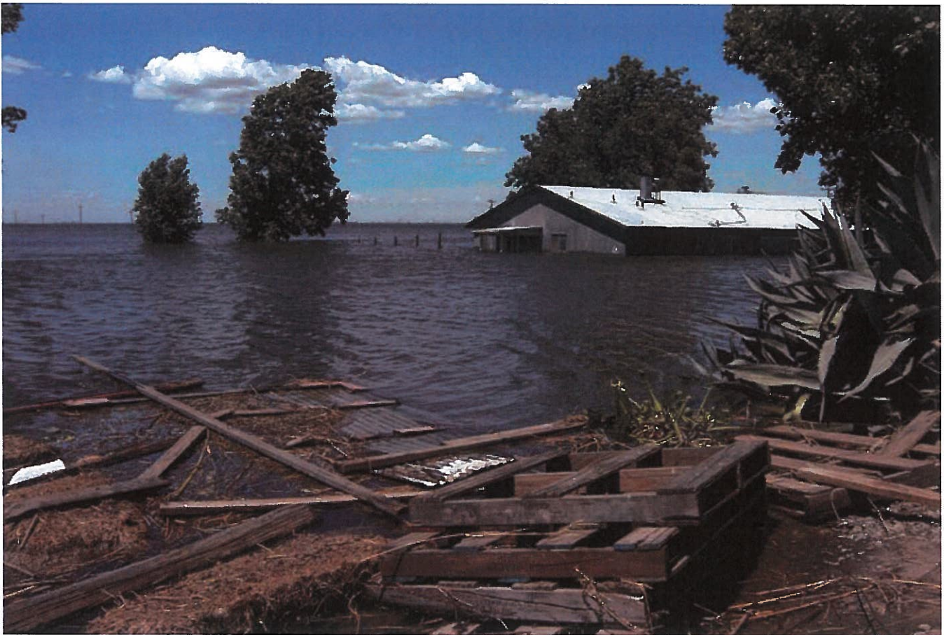
Flood damage – Delta [June 7, 2004]. Source: DWR
