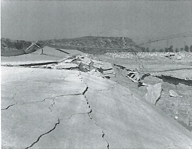
Earthquake damage – Sylmar [February 9, 1971]. Source: DWR
