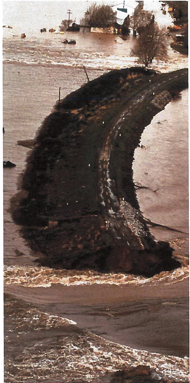
Levee breaches at Tyler Island [1986]. Source: DWR
