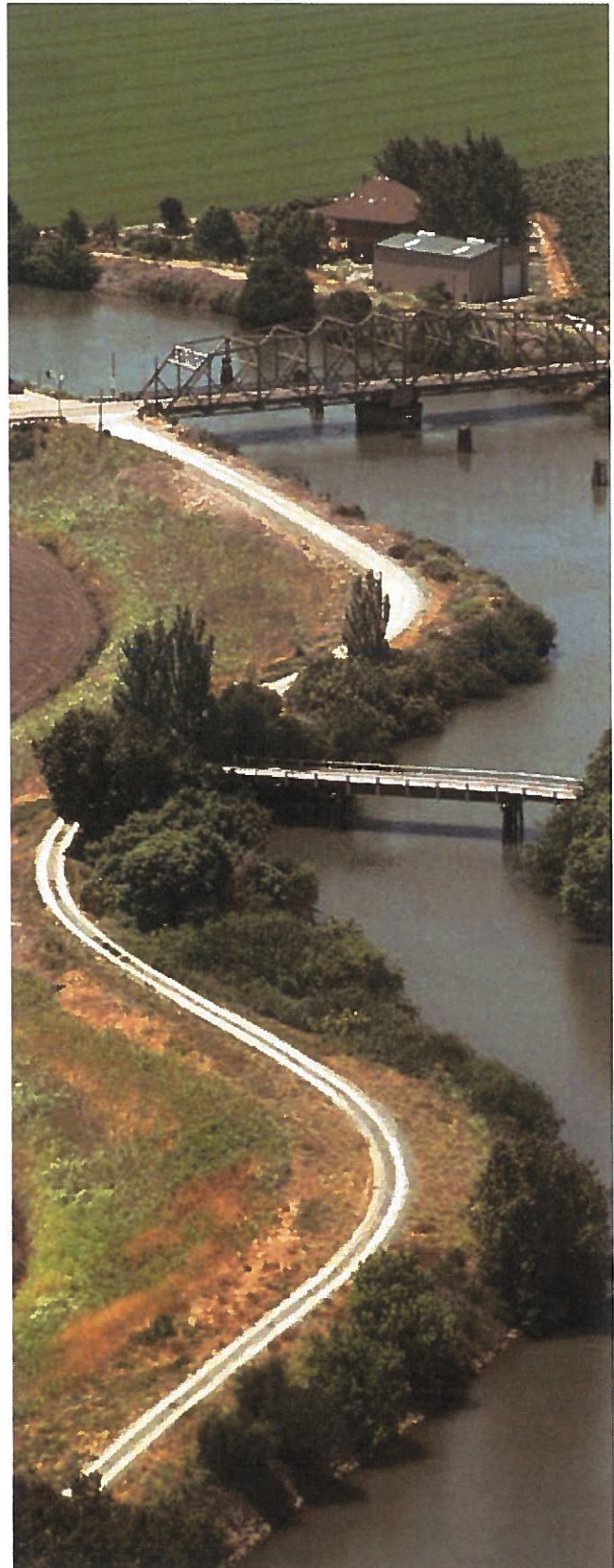
North Walnut Grove Rd. Bridge between Tyler and Staten Islands [larger bridge]. Source: DWR
